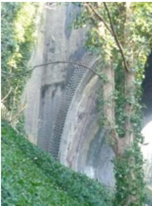
The picture on the left is of the bridge spanning the track-bed of the old St Albans to Hatfield railway line showing the skill of the brick-layers a 100 years or more ago, to create a skewed span using seven layers of bricks. The picture was taken on 30<sup>th</sup> December 2014, whilst Fetes and Fairs ran a train service for the morning along the track-bed.
