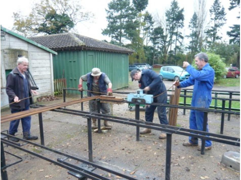
The photo above shows some of the team in action during a working session. The guys are bending rebar into hoops using Gerry's rail-bender machine. These hoops will form part of the reinforced steel work going over Ted's arched brickwork on the GLR tunnel.
